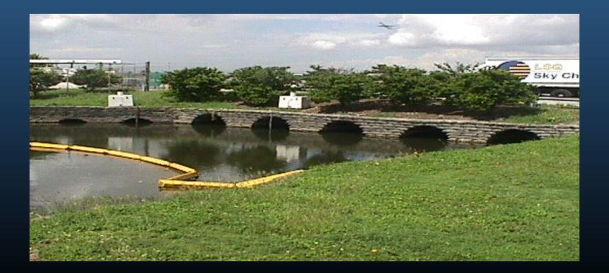
Barriers are installed at outfalls to prevent manatees from entering the drainage system.
